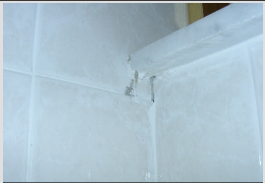
Caulk both ends of shower curb interior
